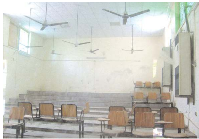
Students share broken wooden chairs as teetering ceiling fans circle overhead
