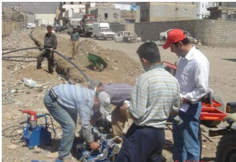
Engineers at a water network expansion project site.
