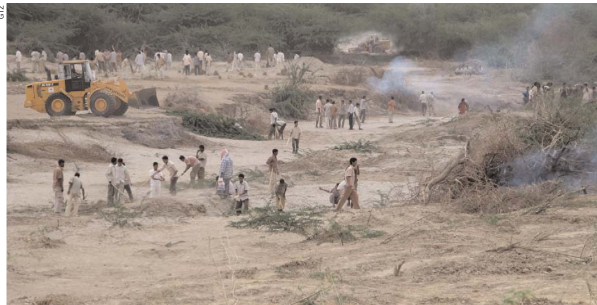
Locals in Abyan removing trees to clear the floods path way in order to prevent flash floods in the area.
