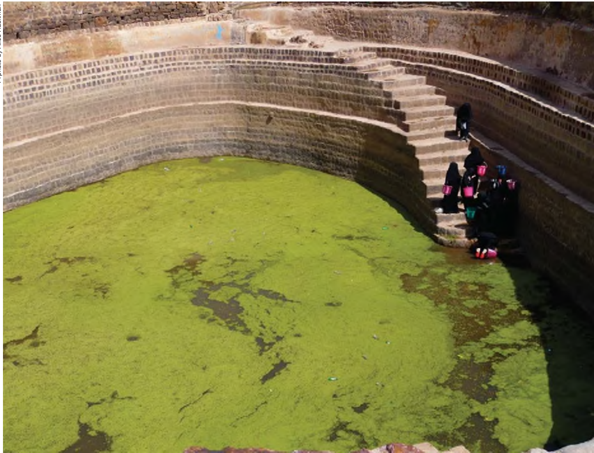
In Shahara, villagers have water piped into their homes, but they still gather water for household use from a traditional rainwater harvesting system.
