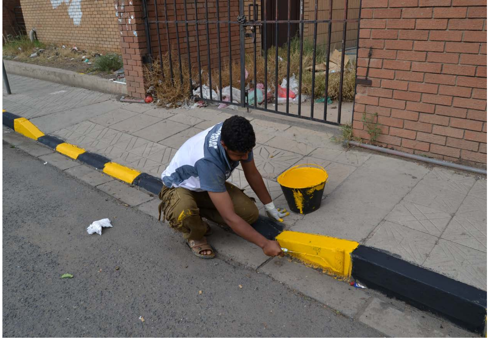
Mohammed Noman works as a painter while studying at university and holding an additional job as a security guard.
