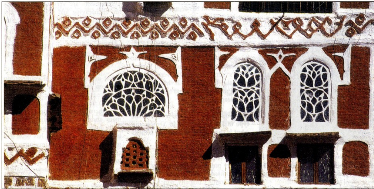
Sana'ani House architecture building
