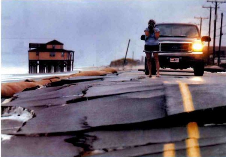
A woman takes video footage of the damaged caused by surging waves to Highway 12 in Kitty Hawk on the Outer Banks of North Carolina, Sept. 18. REUTERS
