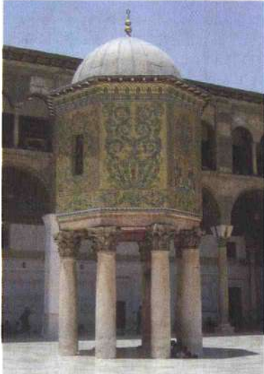
Spectacular erection inside the courtyard
