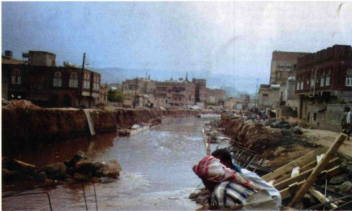
Recent downpour revealed the poorly planned sewage systems which subsided in many areas of the capital city. YEMEN TIMES PHOTO BY WESAM MOHAMMED
