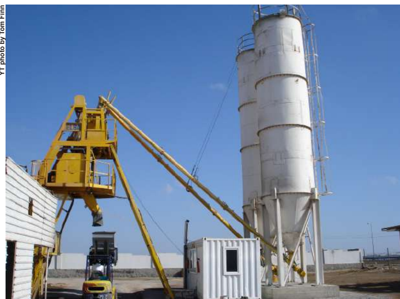
Building the Aden Free Zone.
