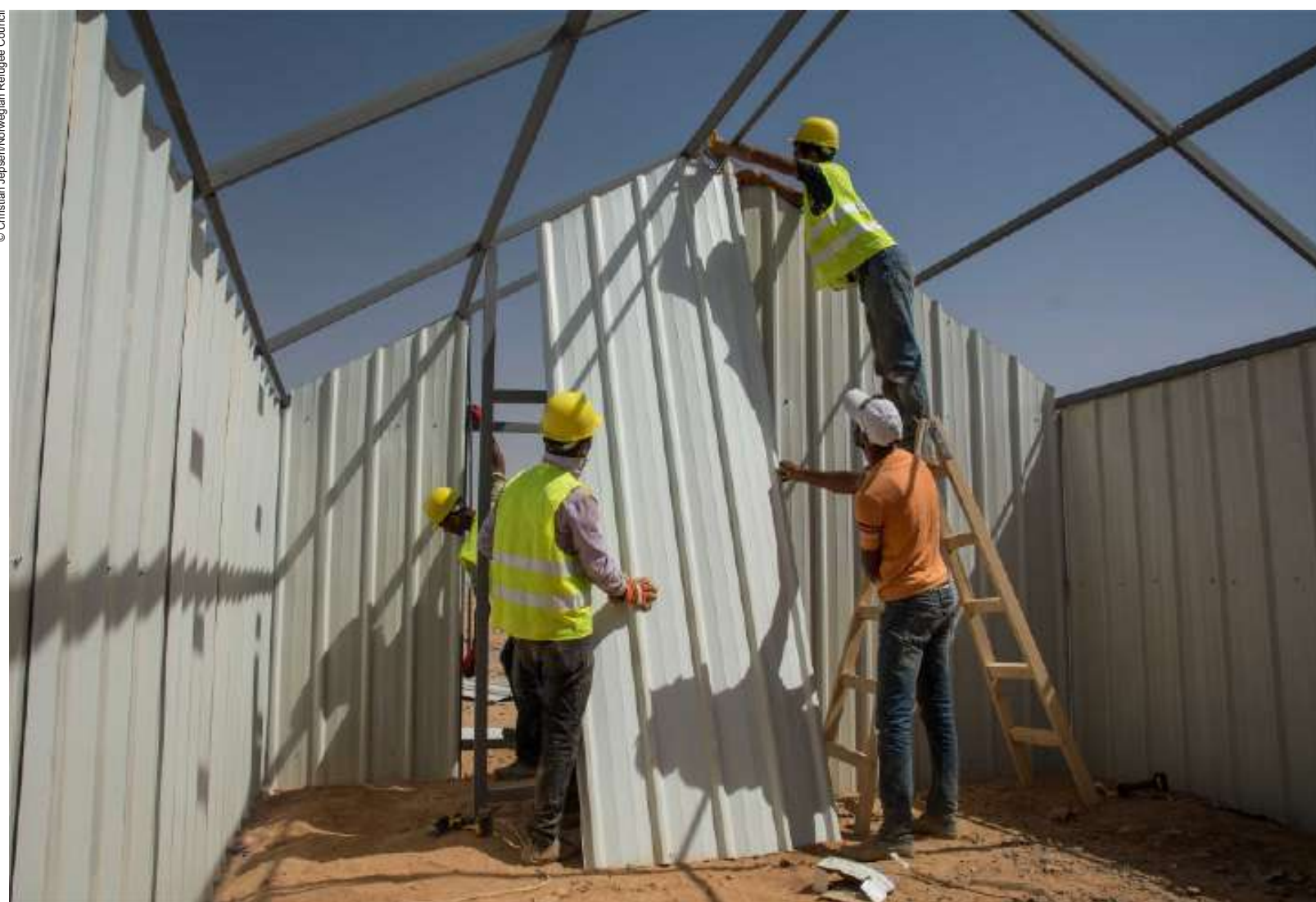
Workers put up specially-designed metal shelters—more resistant to the elements—in Azraq, a new camp for Syrian refugees in the Jordanian desert.
