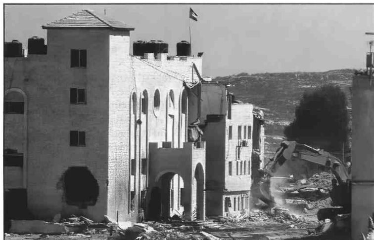
Israeli army continues to destroy buildings at the headquarters of Palestinian President Yasser Arafat in the West Bank City of Ramallah on September 21, 2002, Yasser Arafat vowed not to capitulate to Israel on Saturday after its forces demolished parts of the building where he was under siege and fired a tank shell that showered him with dust. REUTERS
