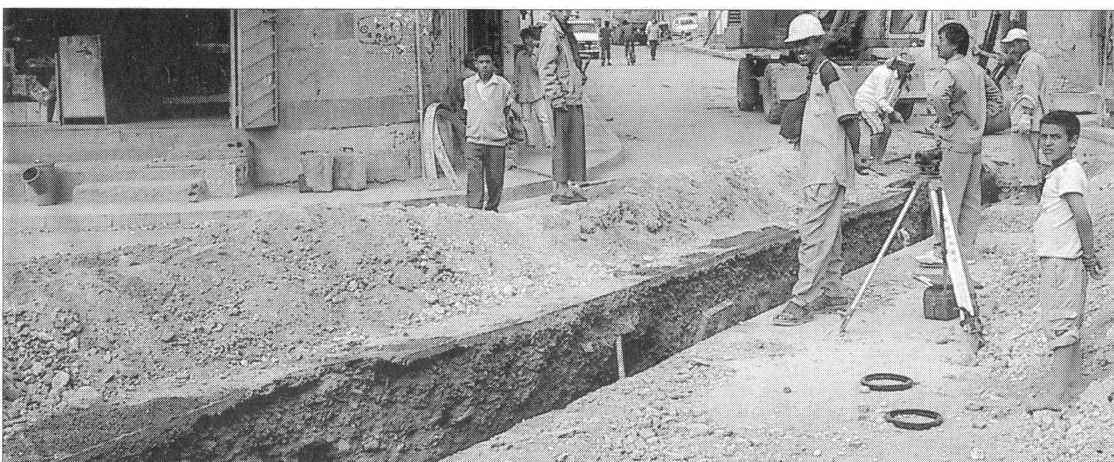
Building water sewerage network
