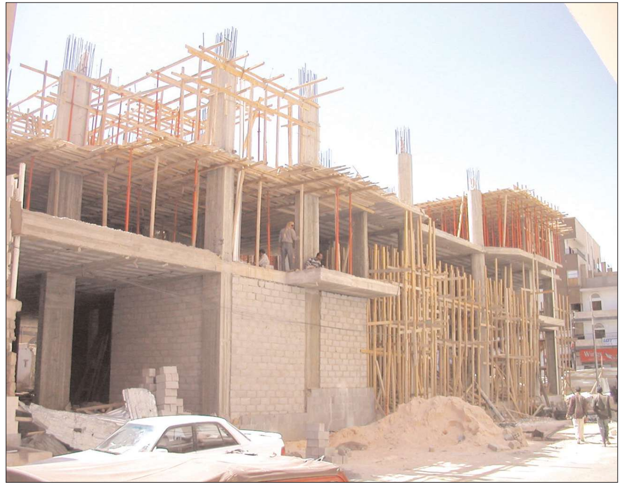
Building of Project under construction.
