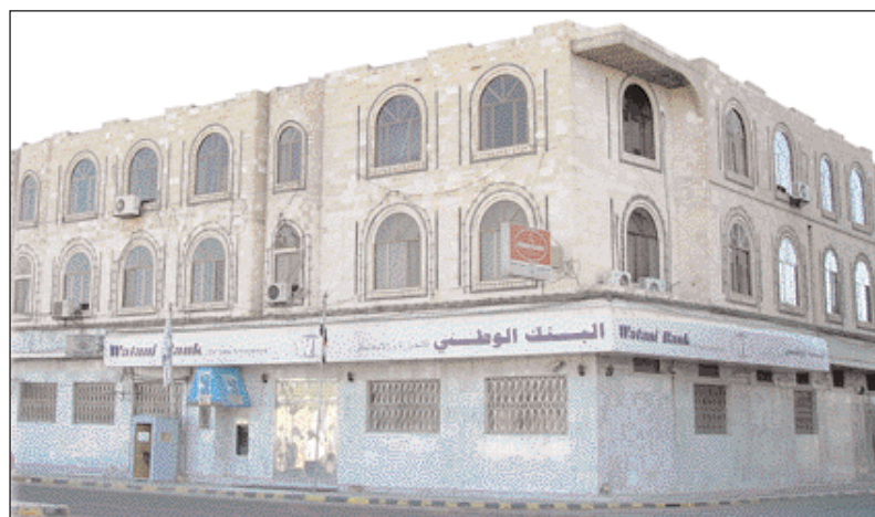
Watani Bank building in Sana'a.
